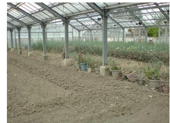
Carnation house damaged by the tsunami
